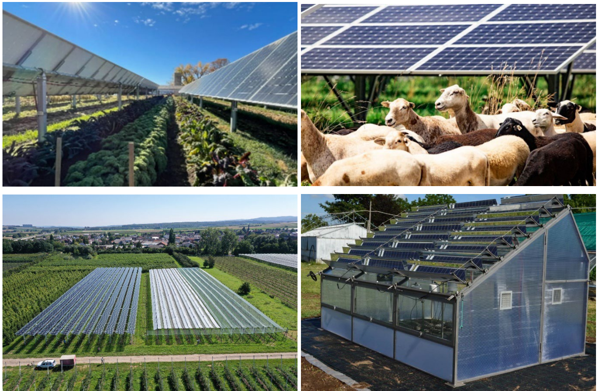
Figure 2. Representative agrisolar system configurations: arable land, permanent crops, pastures, and protected agricultural structures: top left Elevated Crop-PV / Interspace Crop-PV, top right PV with livestock grazing, bottom left elevated perennial-PV/orchard systems, bottom right PV greenhouses
